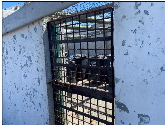
Figure 15. Signal School waste cage.
