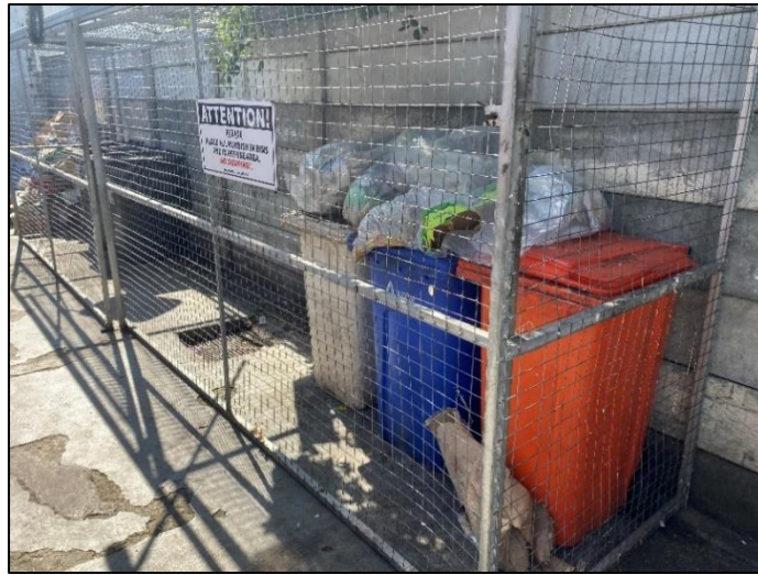
Figure 8. Waste cage at Forest Glade retail centre.
